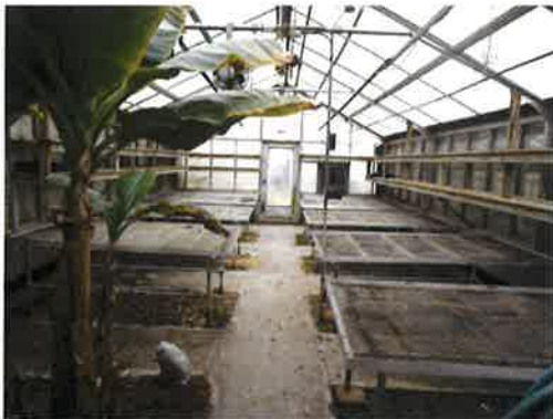
GH#1 - View from retail shop door
