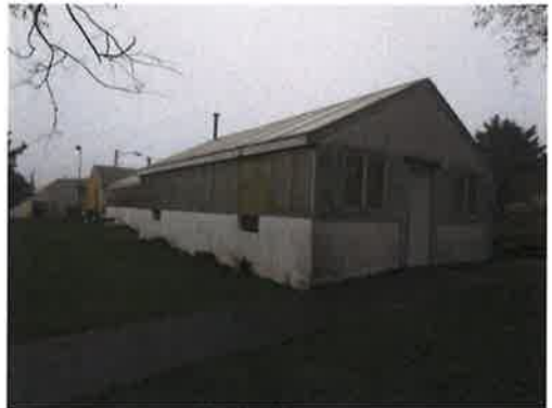
Rear side & Left/rear portion – GH#3 extension
